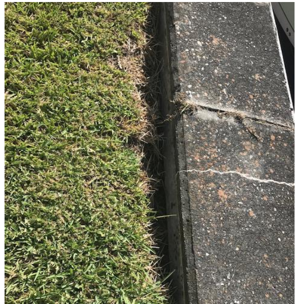
Photo 018 – subsidence, Station 17+30, note soil erosion below the cap flange.
