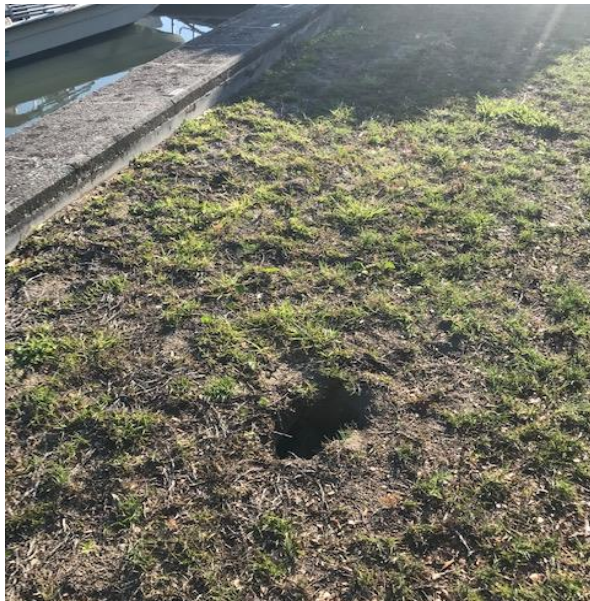
Photo 009 – sinkhole/backfill erosion, the center of sinkhole was about 3 feet from wall, Station 51+55, nearby marker Plate #9
