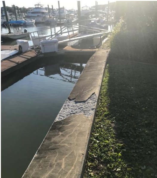
Photo 003 – cap deterioration, exposed aggregate, Station 59+00
