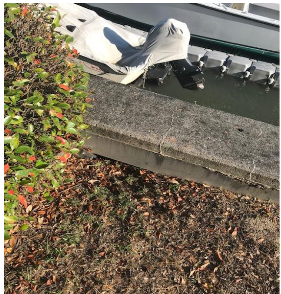
Photo 010 – subsidence, Station 47+55, note shrubs very near the wall.
