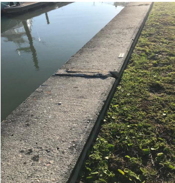
Photo 007- cap joint displacement, Station 56+00
