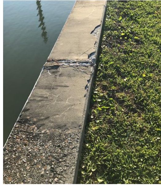
Photo 002 – Cap deterioration/concrete spalling, Station 59+30
