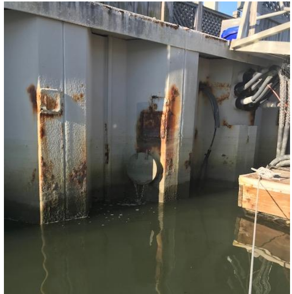
Photo 008 – Flapper valve, functioning mid tide
