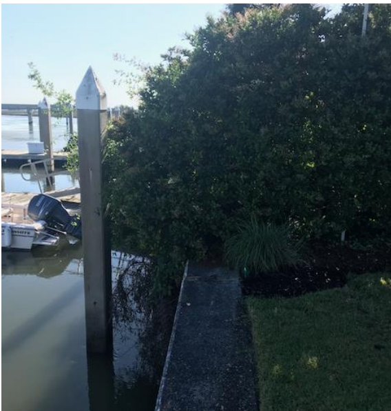
Photo 015 – Trees and shrubs have been planted very near to back side of the wall. The wall cap has completely been covered by overgrown shrubs and trees, Stations 30+70 to 33+00, typical
