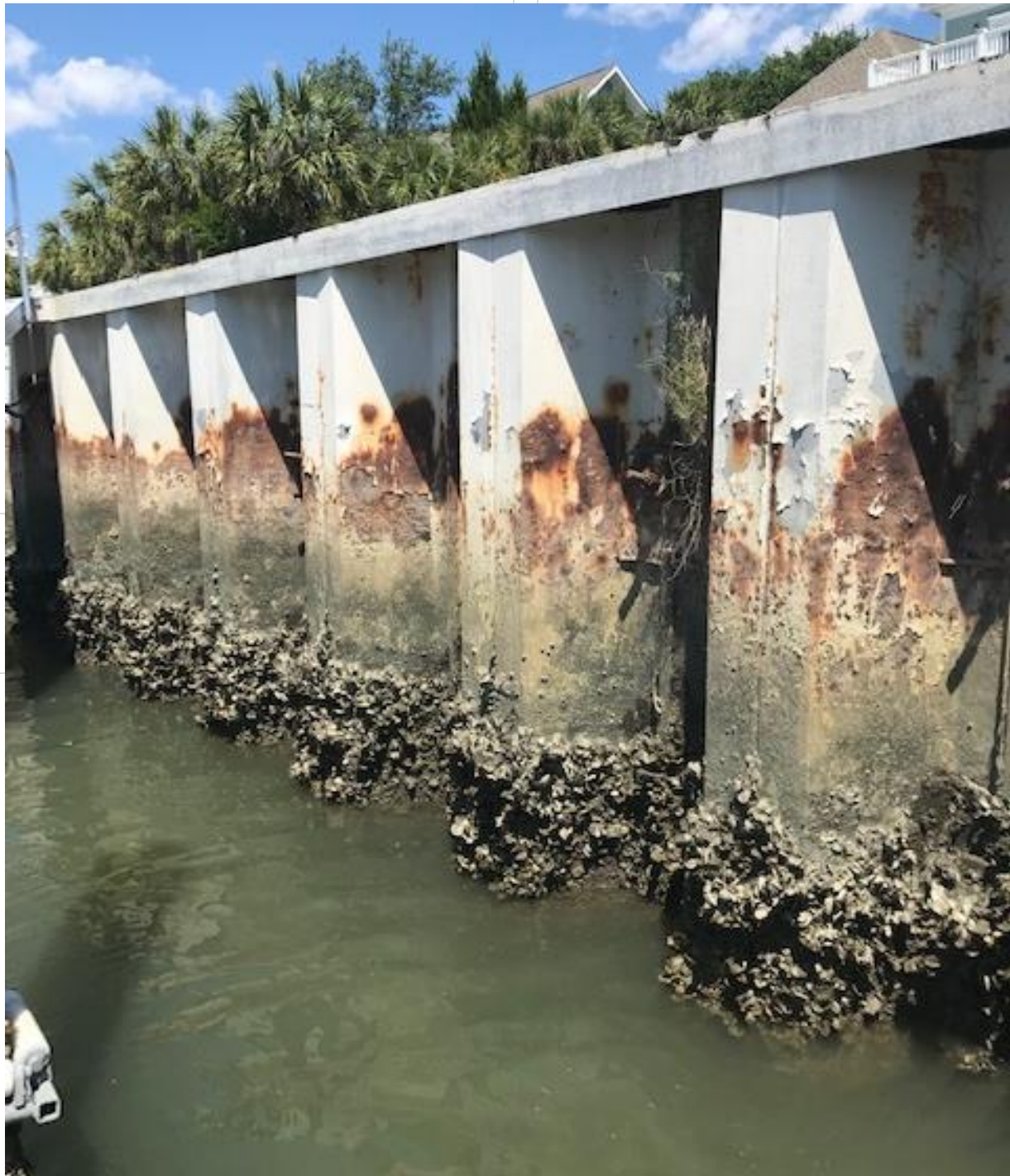
Photo 021- typical corrosion and marine build up. Note rust on anchorage assembly.
