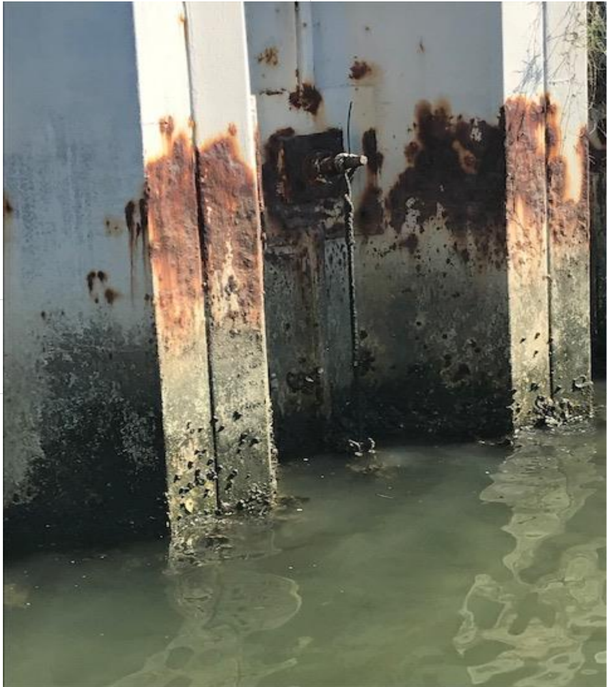
Photo 022 – corrosion on wall and anchorage assembly.
