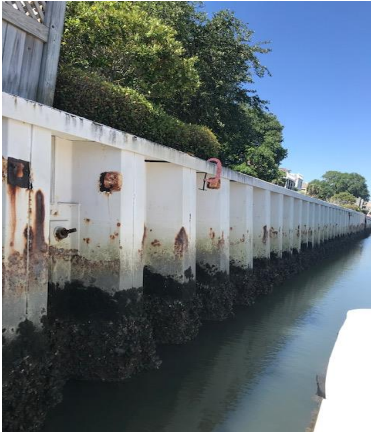
Photo 020- typical corrosion and marine build up. Note rust on patch plates. Also, numerous pinholes.
