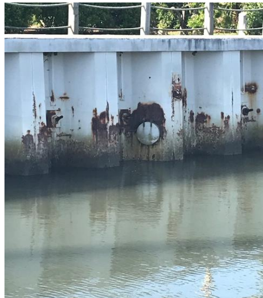
Photo 012 – rust/corrosion (typical) around flapper valve, anchorage and bulkhead, Station 45+50
