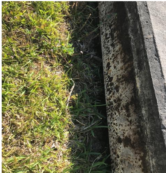
Photo 019 – subsidence, Station 22+25, deep erosion below cap.
