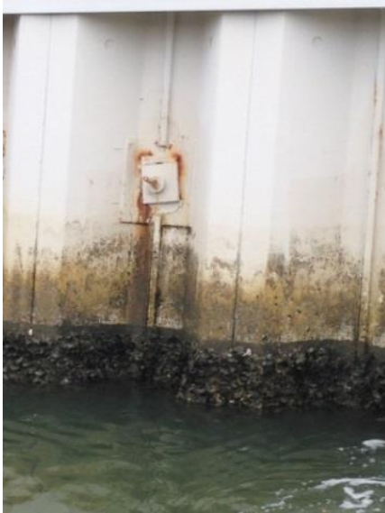
Photo #11 – Anchor slippage as reported in past inspections
