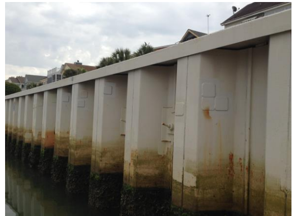
Photo #2 – Minor rust adjacent to patch plates, but overall look good
