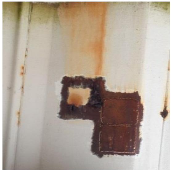
Photo #6 – Closer view of pinholes. The area has been prepared, but patch plate has yet to be placed. G-dock
