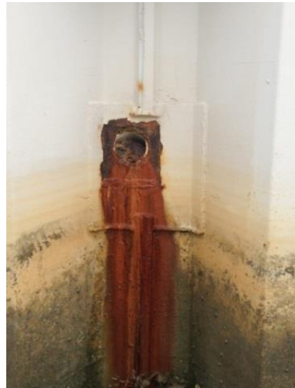
Photo #10 – Missing anchor at 47 Water Way
