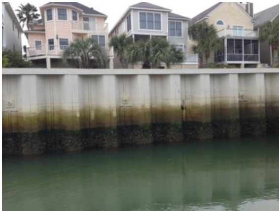
Photo #1 – Typical wall condition where pinholes have been repaired and area re-coated
