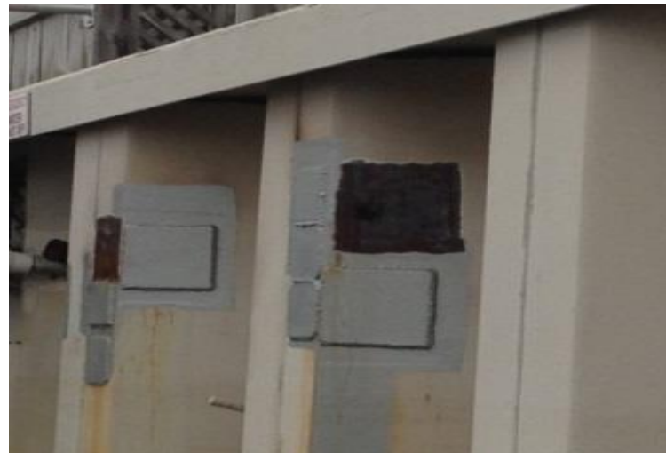
Photo #4 – Same as Photo #3. Additional pinholes adjacent to previously repaired pinholes.
