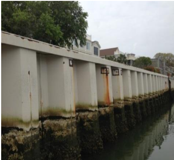
Photo #5 – Pinholes to be patched.
