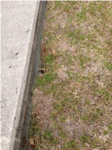
Photo #13 – Backfill subsidence near marker 48+50
