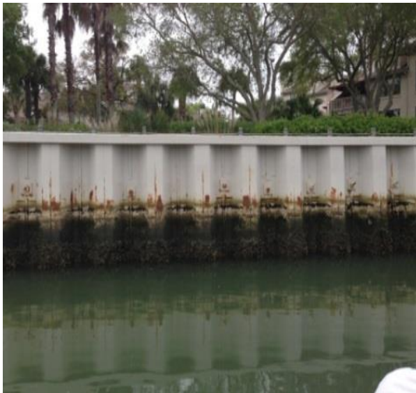
Photo #7 – Wall condition between G and H Docks. Some rust. Pinholes have formed, but have yet to be repaired.
