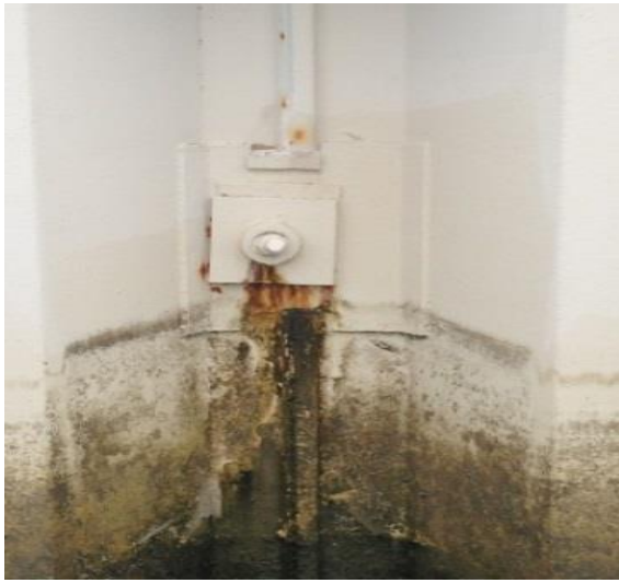
Photo #9 – leaking anchor near marker 38+39
